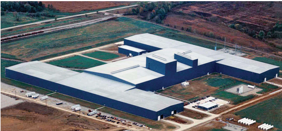
← Heartland Steel This three-phased industrial complex has 17 acres under roof, using over 6,500 tons of steel.
